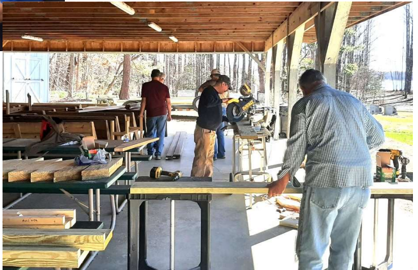
Building New Benches March 18 th
